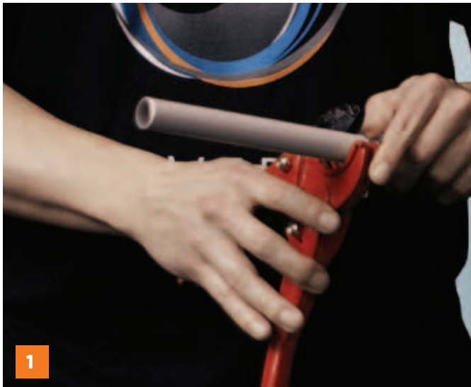
Proper pipe cutting with a cutter
